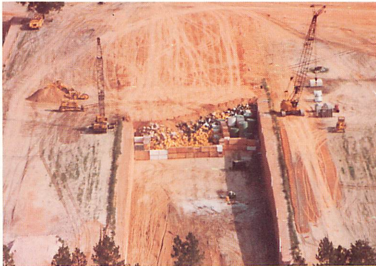
Low-level radiation disposal site in Barnwell, South Carolina.
