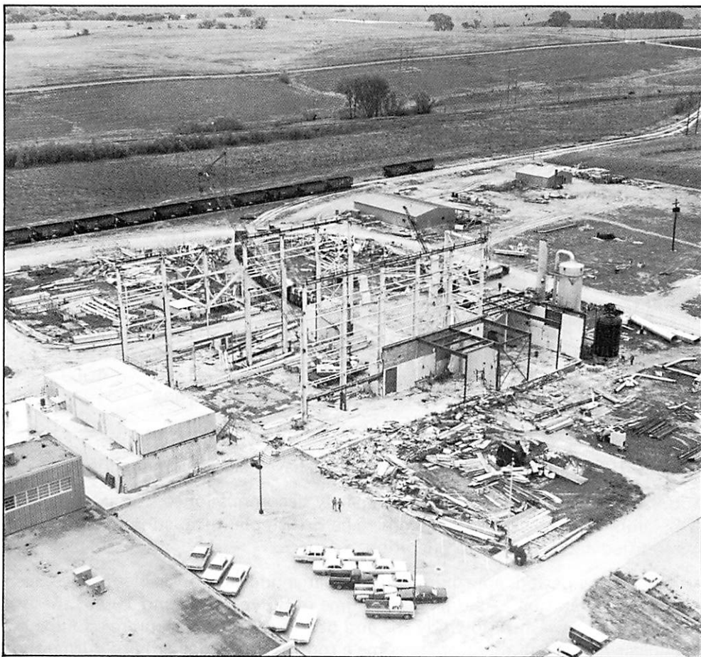
Figure 4. The Hallam reactor in the USA was decommissioned to Stage 2; the work is shown here nearing completion. (Photo: Rockwell International)
